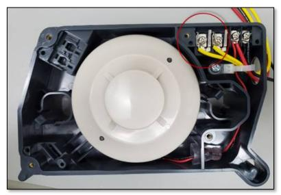
**Figure 1. Smoke Detector Cover**
